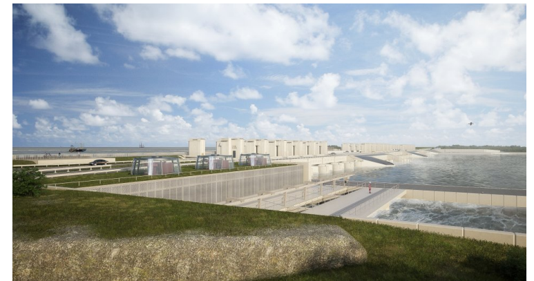
Reinforcing the largest dam in the Netherlands with BIM
